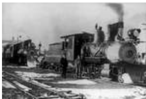
- Special to the Daily/Breckenridge Heritage Alliance
